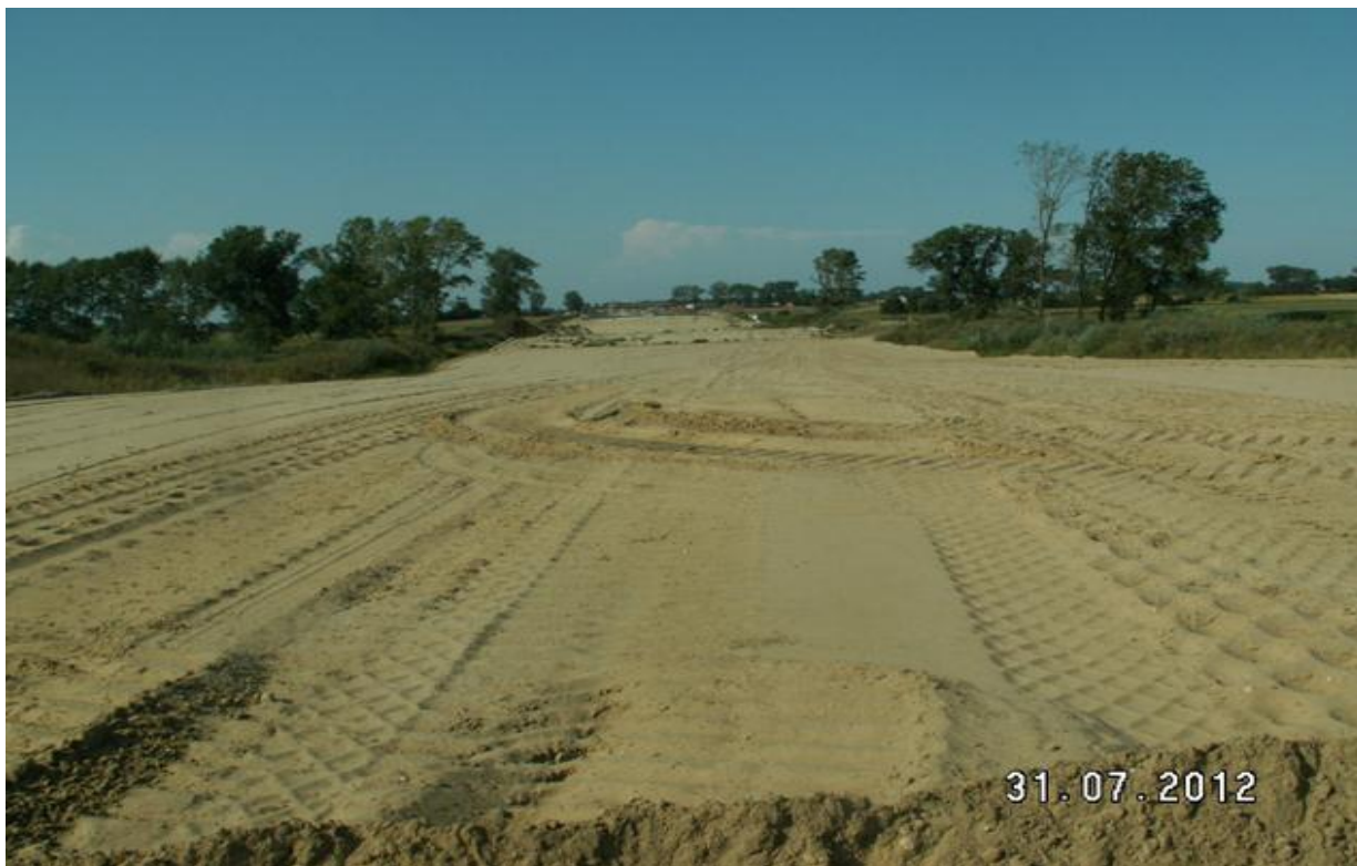
Nasyp z dokopu km 259+150-259+350
